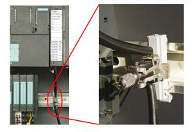
Figure 6.5: Connecting the cable shielding to the PLC
