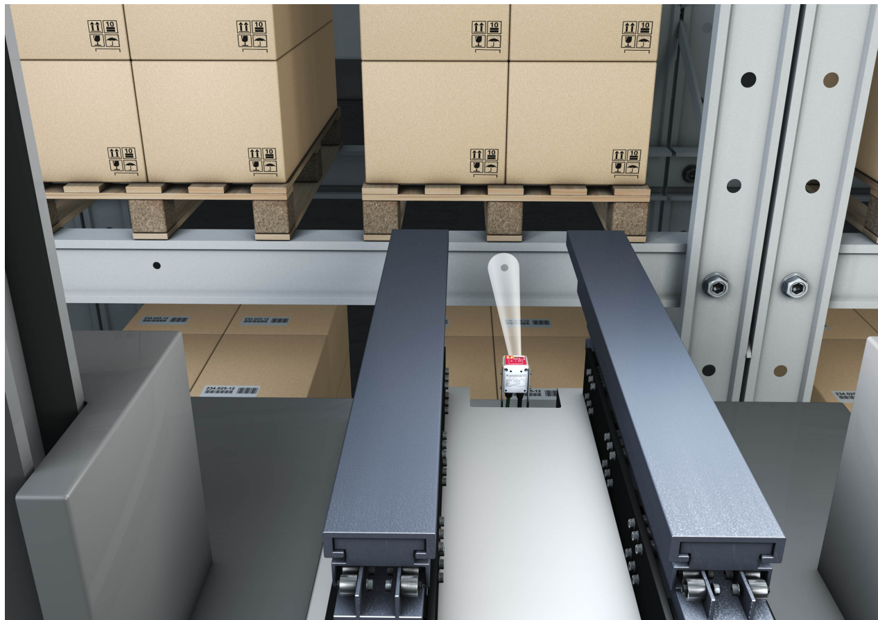
Fig. 5.1: Compartment fine positioning of a high-bay storage device in a single-depth high-bay pallet warehouse
