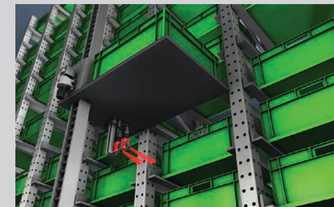
Positioning in container warehouse
